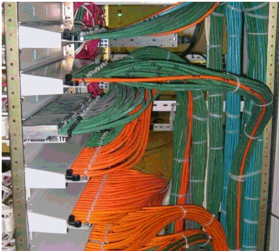
Figure 4.3 – Example of wiring in a distribution box
